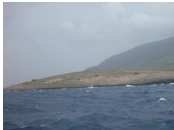
Entry to the bay of Vlora plenty of bunkers
